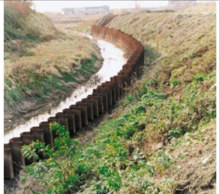
Ref: Northern Sheet Piles Ltd (work in progress)
